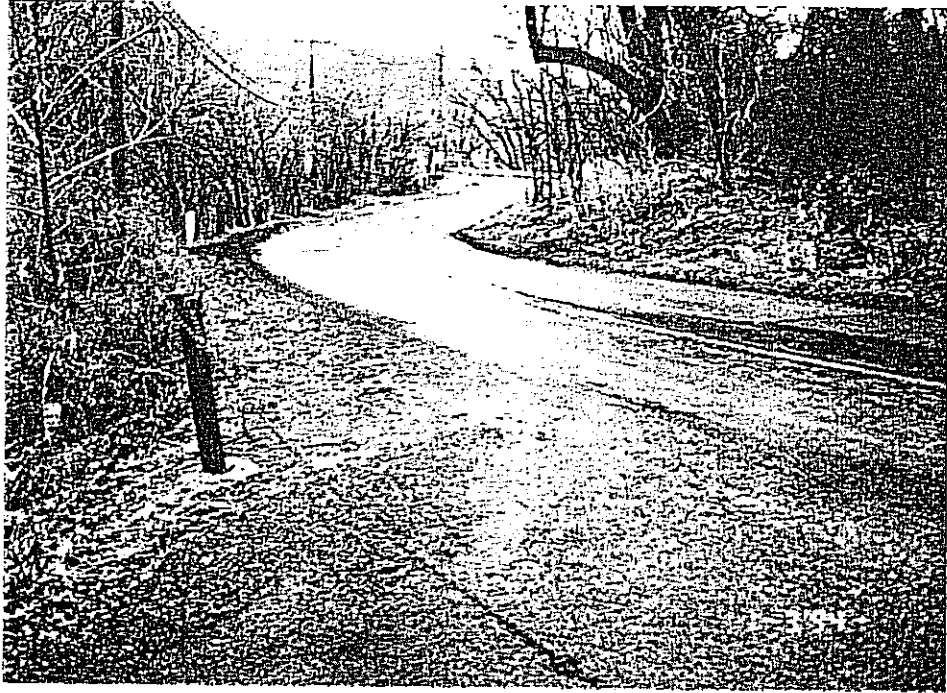
Picture of the Dreman Avenue roadway and the east approach to the bridge. Notice the poor roadway alignment and the unimproved roadway conditions. Picture taken from Dreman Avenue looking northwestward.
