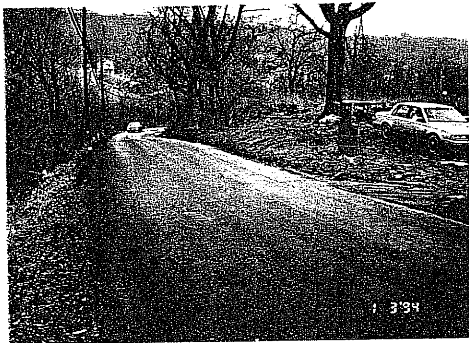
Picture of the Dreman Avenue roadway. Notice the unimproved roadway conditions. Picture taken from near the Beekman Street intersection looking westward.
