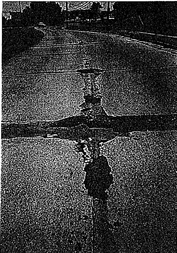
TYPICAL HIGH SEVERITY TRANSVERSE JOINT FAILURE. TYPICAL MEDIUM-HIGH LONGITUDINAL JOINT FAILURE. NOTE THAT THERE ARE TWO TRANSVERSE CRACKS THAT RUN COMPLETELY ACROSS THE PAVEMENT BEFORE THE NEXT JOINT. THIS IS TYPICAL DUE TO THE SPACING BETWEEN JOINTS, WHICH AVERAGES 50 FEET.
