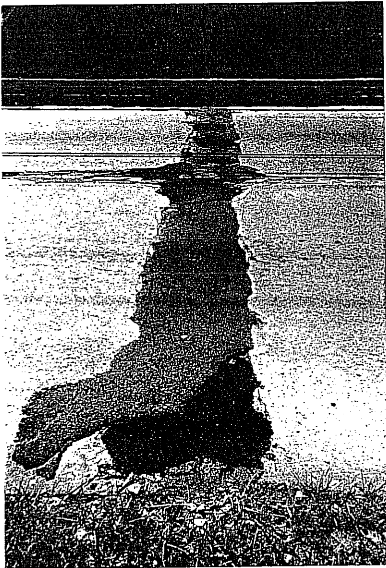
THE CONCRETE PORTION OF MANGHAM DRIVE HAS SEVERE JOINT FAILURE ALONG THE CENTERLINE, AND ALSO AT THE TRANSVERSE JOINTS. THE JOINTS HAVE BEEN REPAIRED SEVERAL TIMES.
