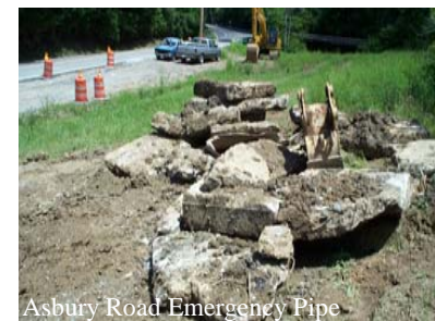
Asbury Road Emergency Pipe
