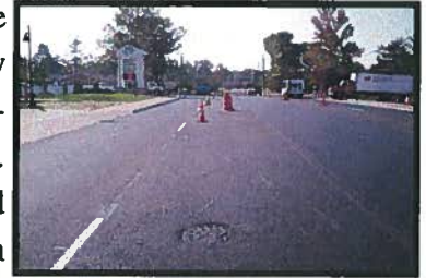
Winton Road Resurfacing
