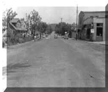
At Grace Avenue looking north
