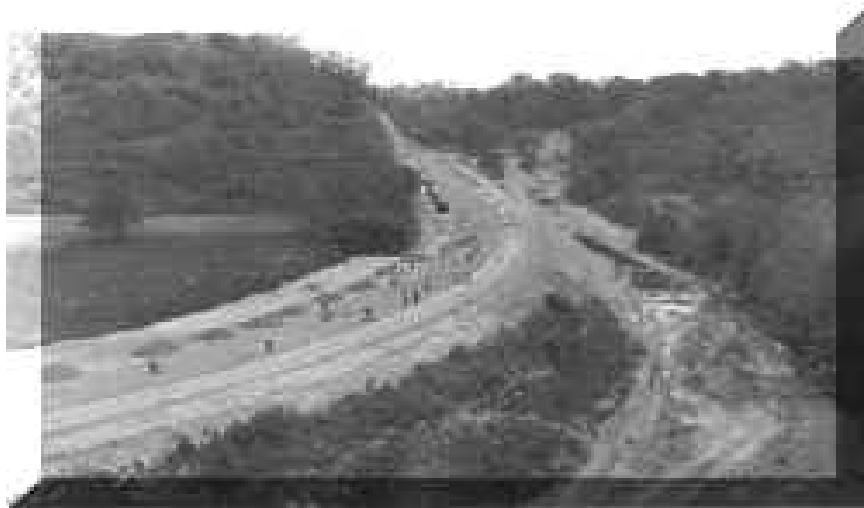
Muddy Creek Road Construction - May 24, 1937 Looking down from Devil's Backbone Road
