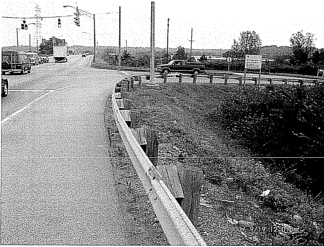
Guardrail at GE Drive
