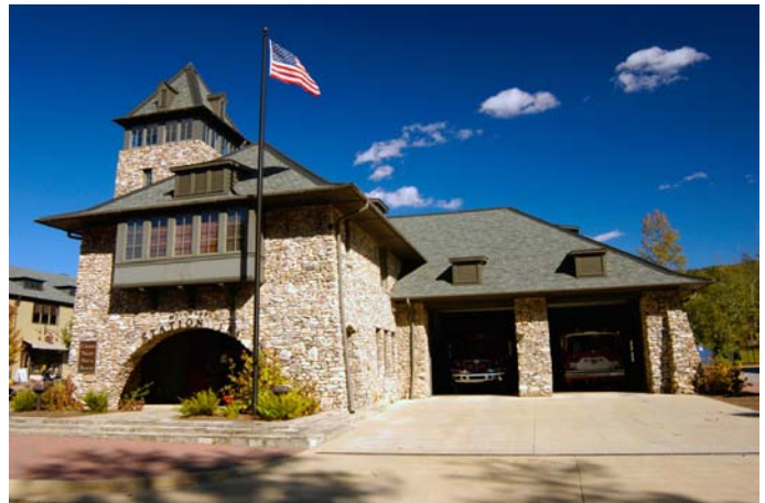
Photo: Fire Station in Mt. Laurel, Alabama features high quality materials and design
