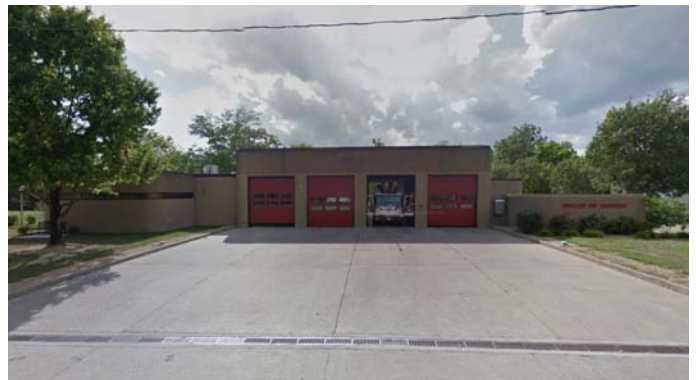
Photo: Existing Fire Station
