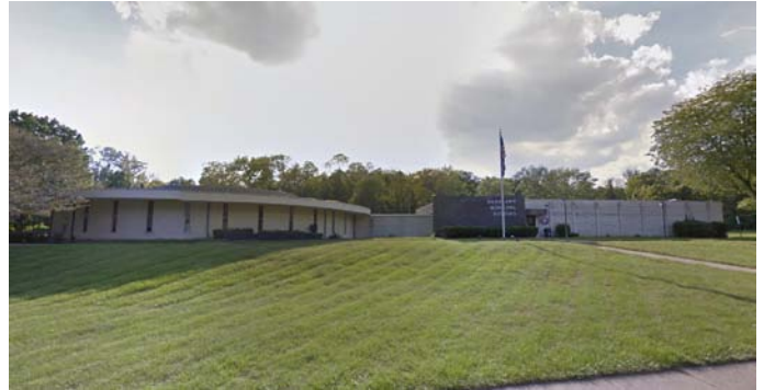
Photo: Existing Public Administration & Police Headquarters Building
