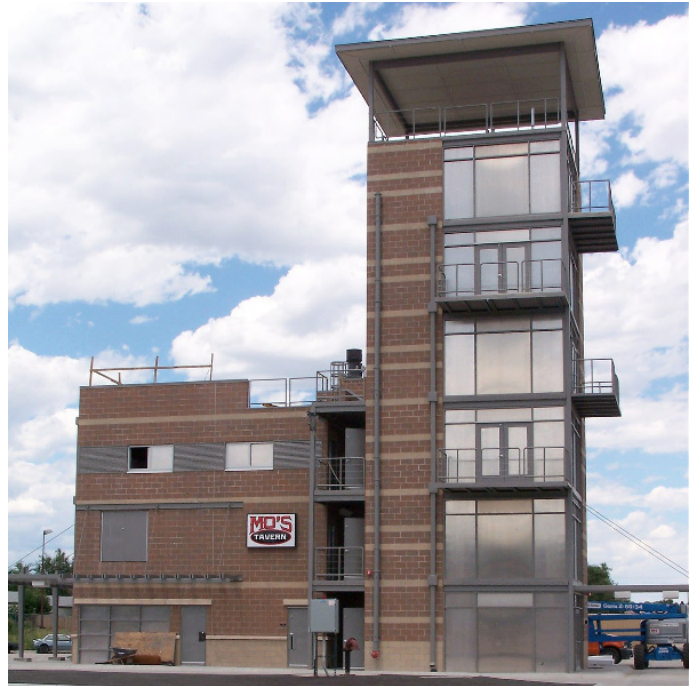
Photo: Fire Training Tower can also serve as a community wayfinding marker
