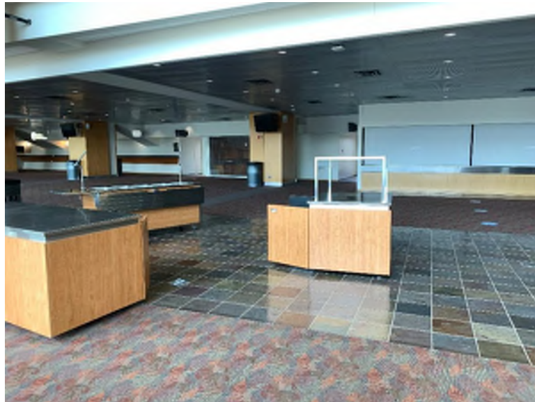
Club space showing broadloom carpeting and slate tile flooring and movable food stands. The back of photo shows the unused countertop areas on the left, a satellite retail space with a gate in center and a concession stand on right.
