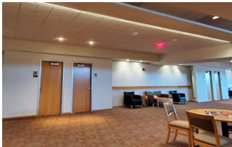
Club corridor lighting
