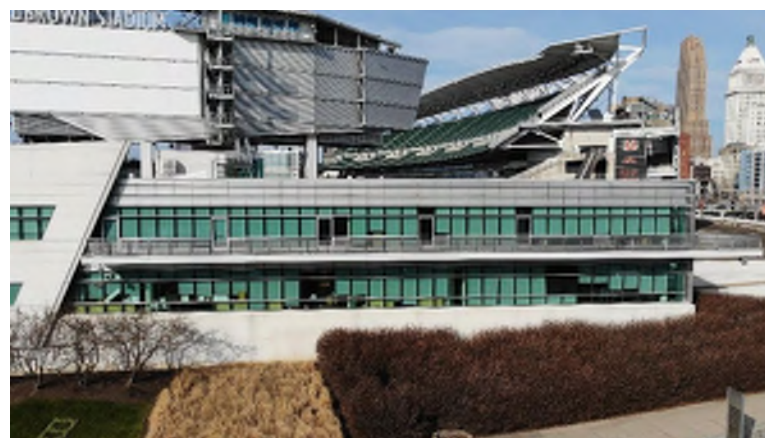
Street side of the Administration Building
