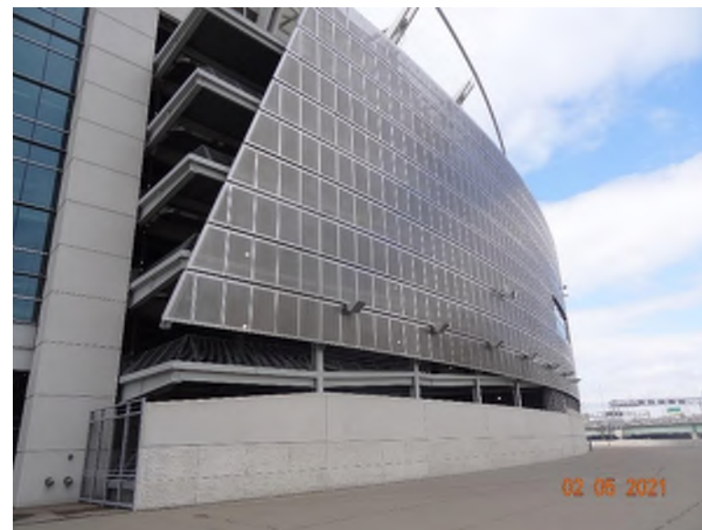
Perforated metal panel screen wall
