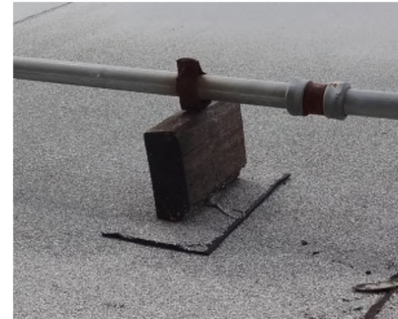
Close up of wood blocking support
