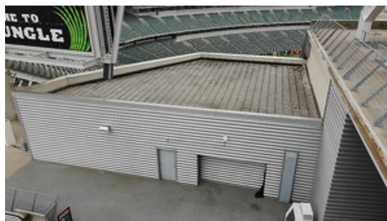
Protected membrane roof
