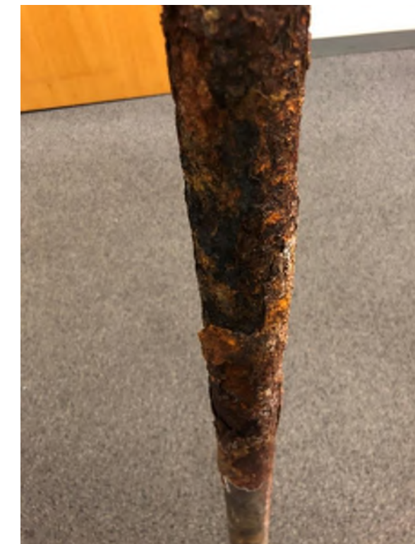
Sprinkler pipe removed and replaced above Bengals Weight Room.
