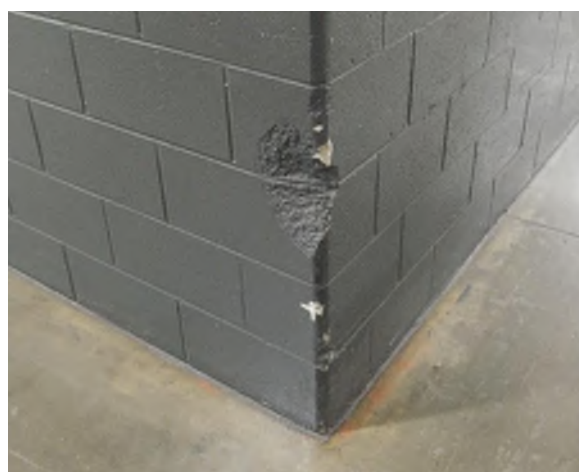
Typical condition of CMU wall corner
