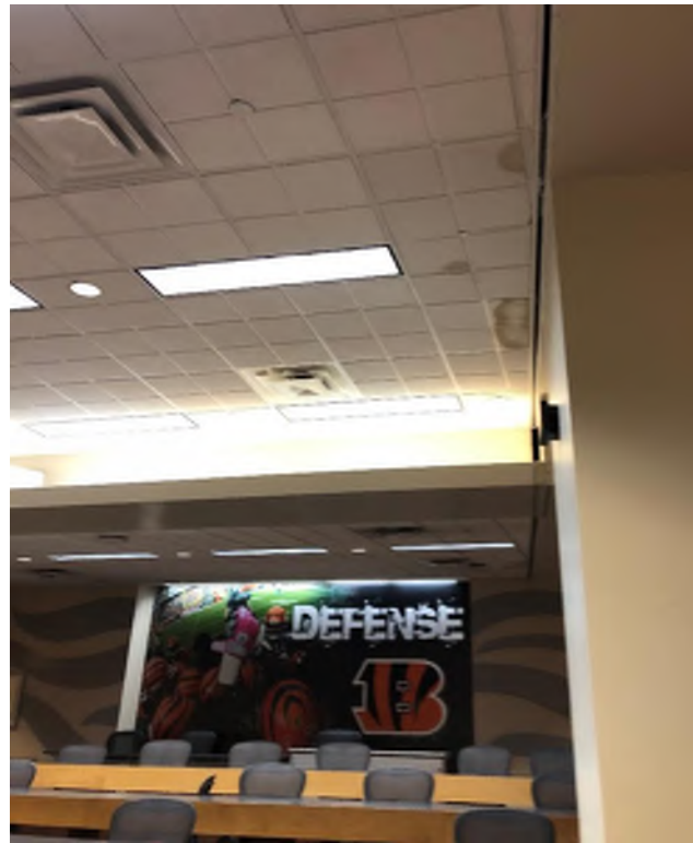
Small Auditorium ceiling.
