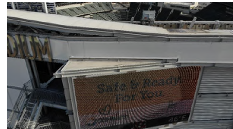
Wedge roof at north scoreboard
