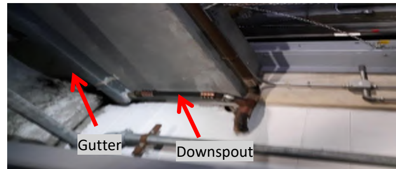
Gutter and downspout
