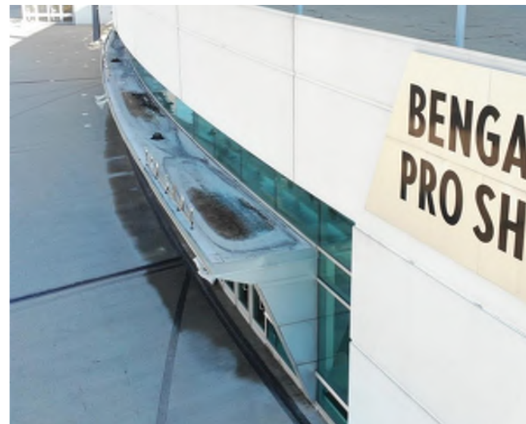
Roof at north ticket window and pro shop
