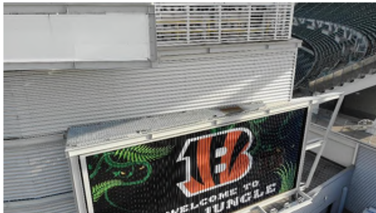
Wedge roof at north scoreboard
