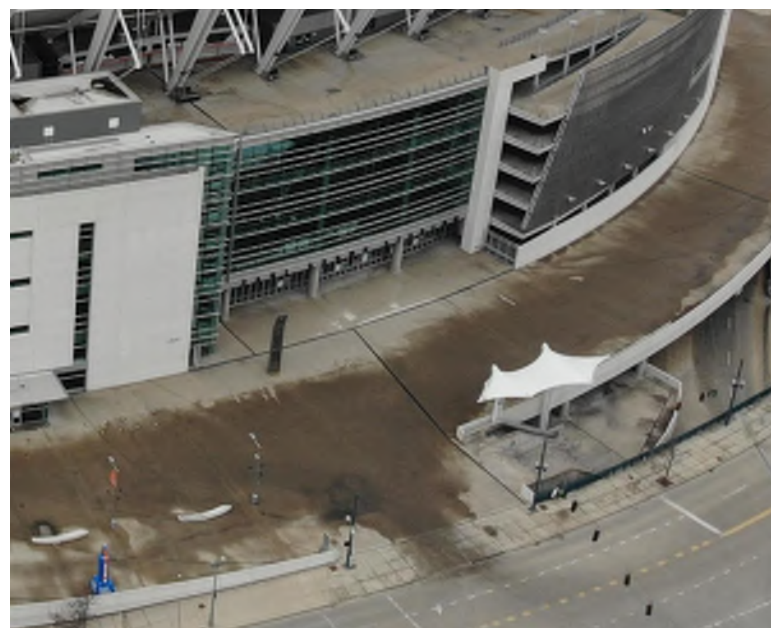
East Exterior Plaza - Gate D and automobile entrance
