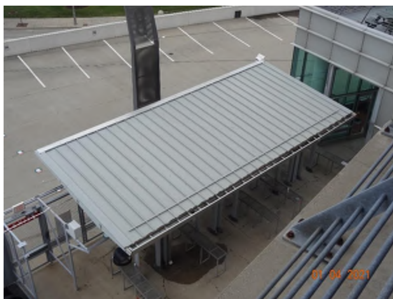
Standing seam roof at gate
