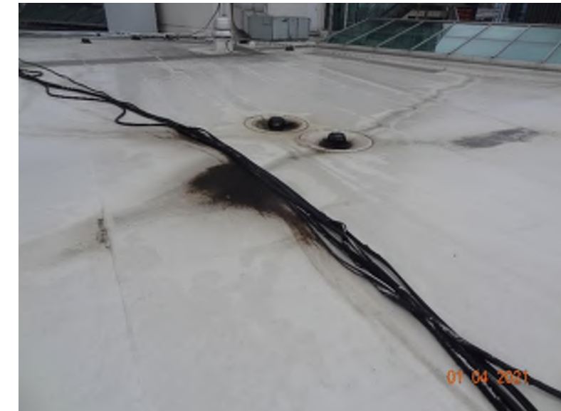
Administration Building – cable on roof
