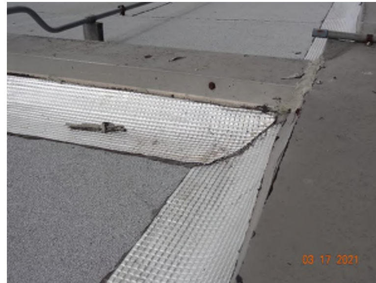
New roof over original metal coping
