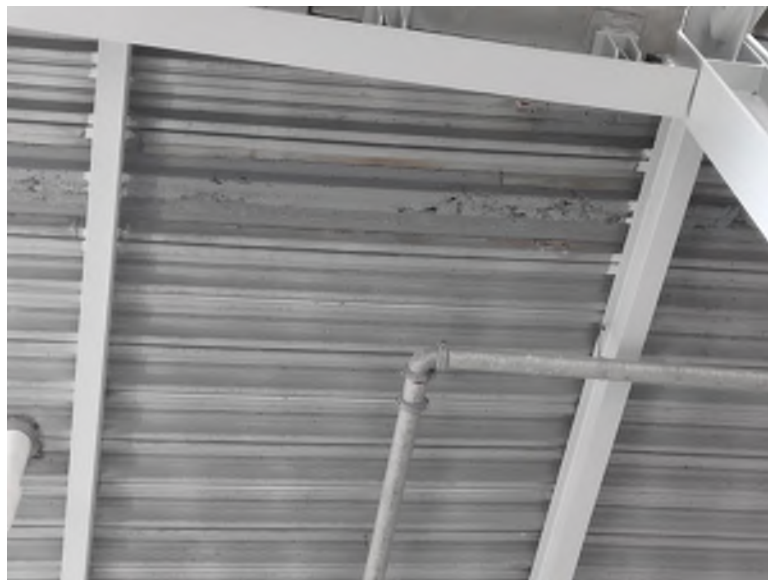
Metal deck after replacement
