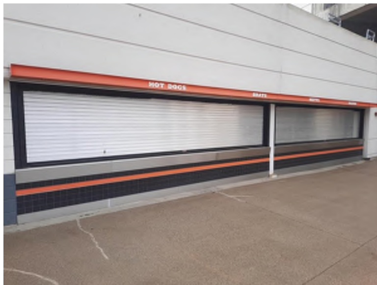
Overhead door after replacement
