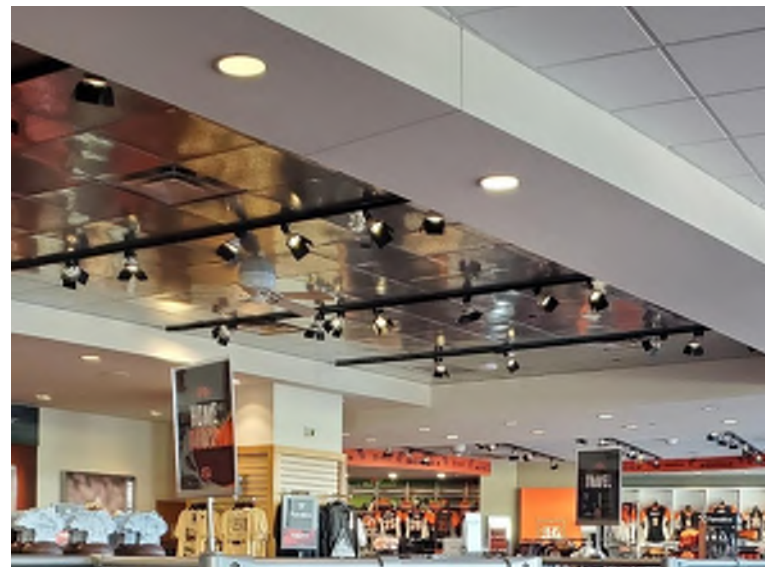
Pro Shop lighting
