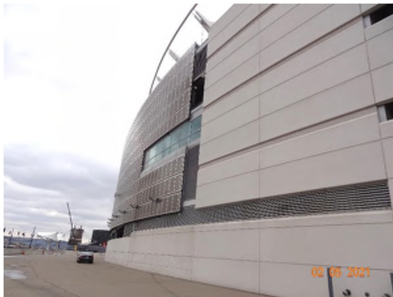
Precast concrete wall panels – stadium exterior
