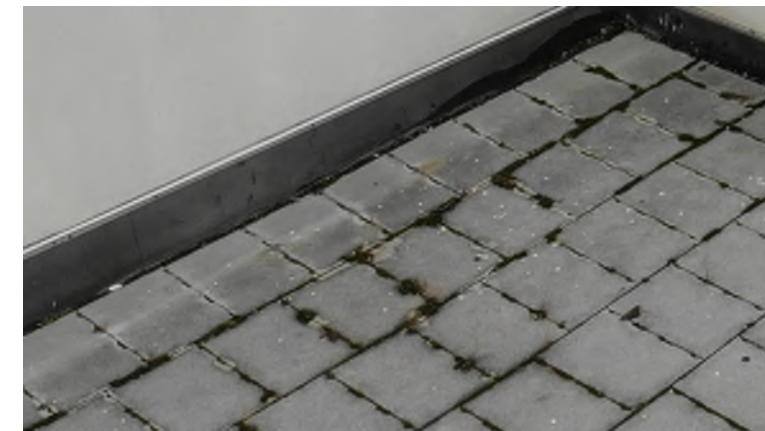
Close-up of protected membrane roof
