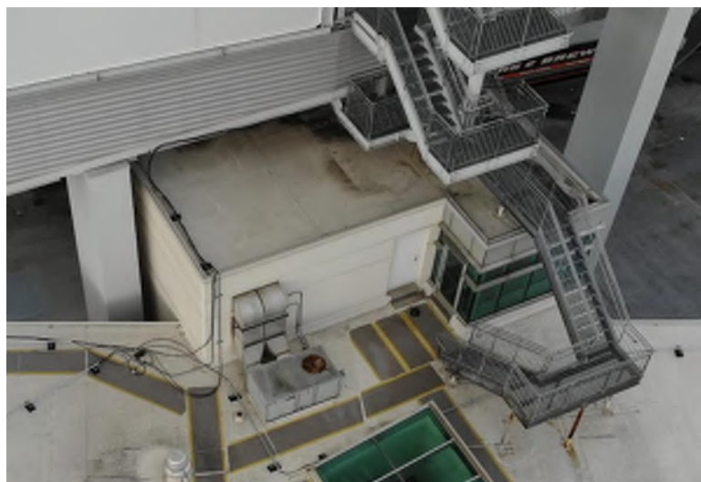
Administration Building elevator roof
