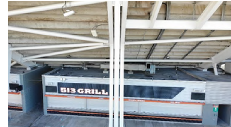
700 level - Concession roof
