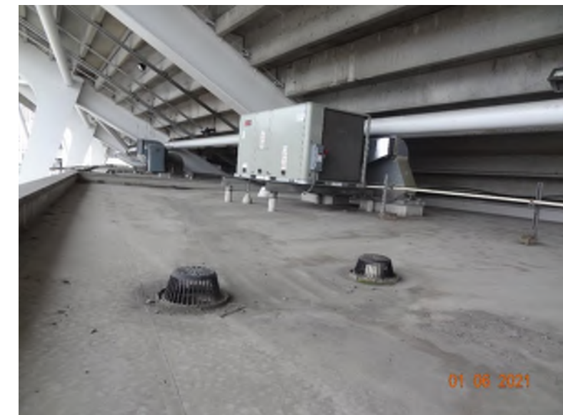
Typical EP membrane roof
