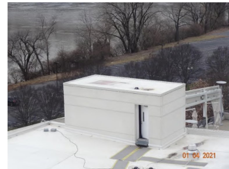
Administration Building – west stair roof
