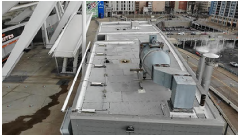
Typical modified bitumen roof
