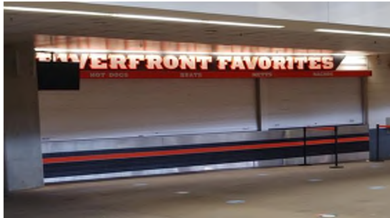
Typical concourse low ceiling fluorescent linear lighting
