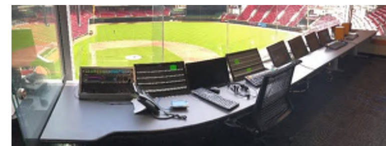
Typical window wall console at Great American Ballpark
