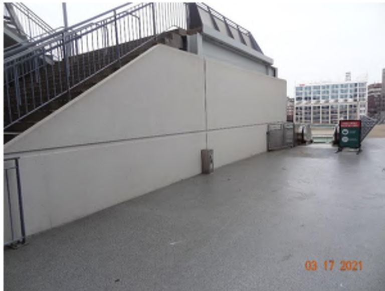
Precast concrete wall panels – concourse walls
