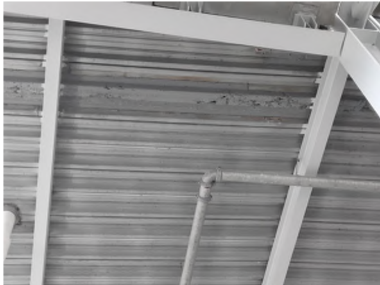
Metal deck after replacement
