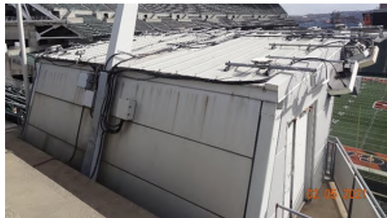
Camera booth roof, typical
