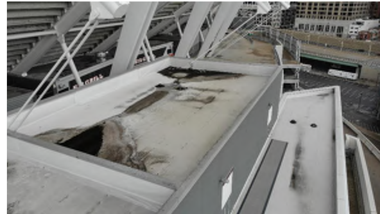
Outer Sector: typical EP membrane roof
