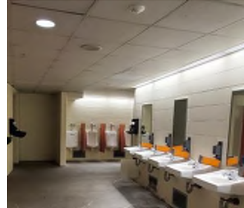
General restroom lighting
