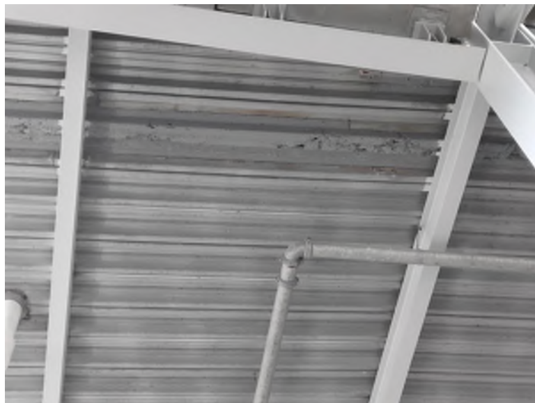
Metal deck after replacement
