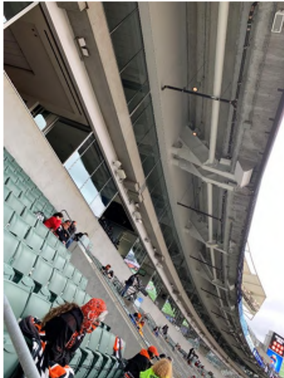
Loudspeaker located under the upper bowl precast overhang serve the lower deck.
