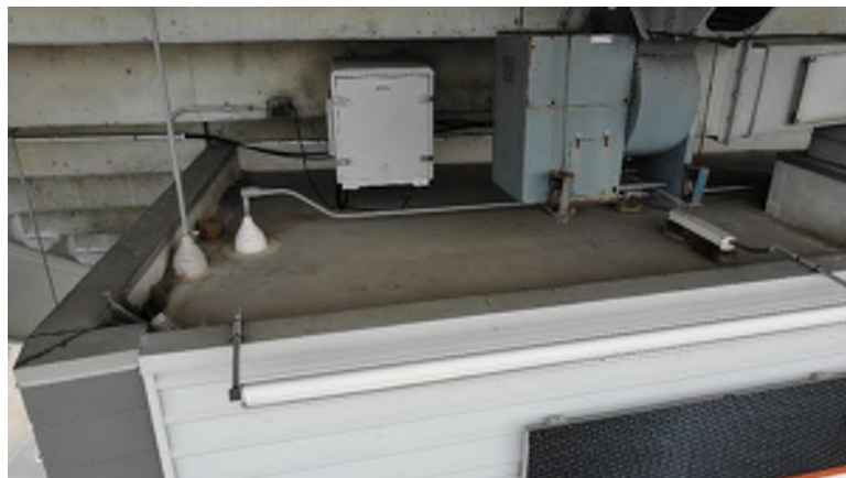
Equipment on roof near roof edge
