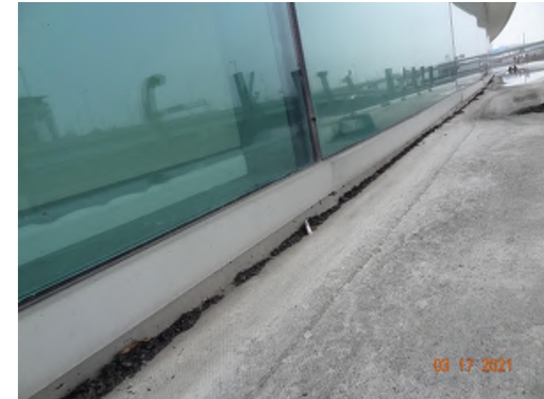
Glazing above pro shop roof
