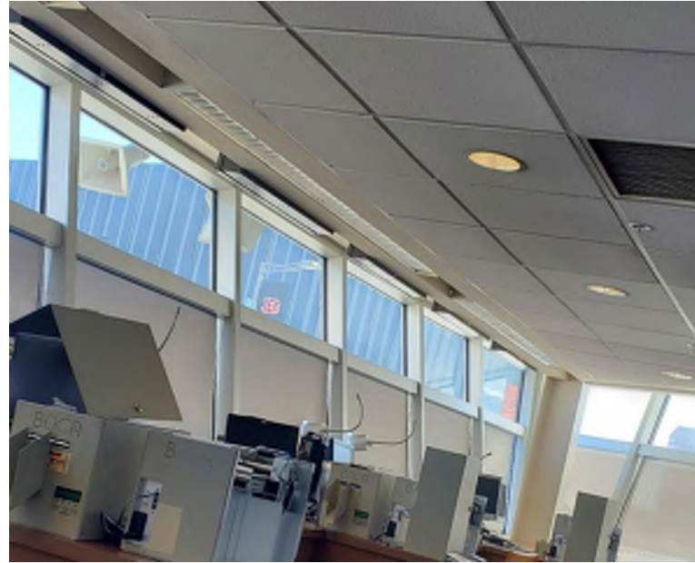
Ticketing Office lighting
