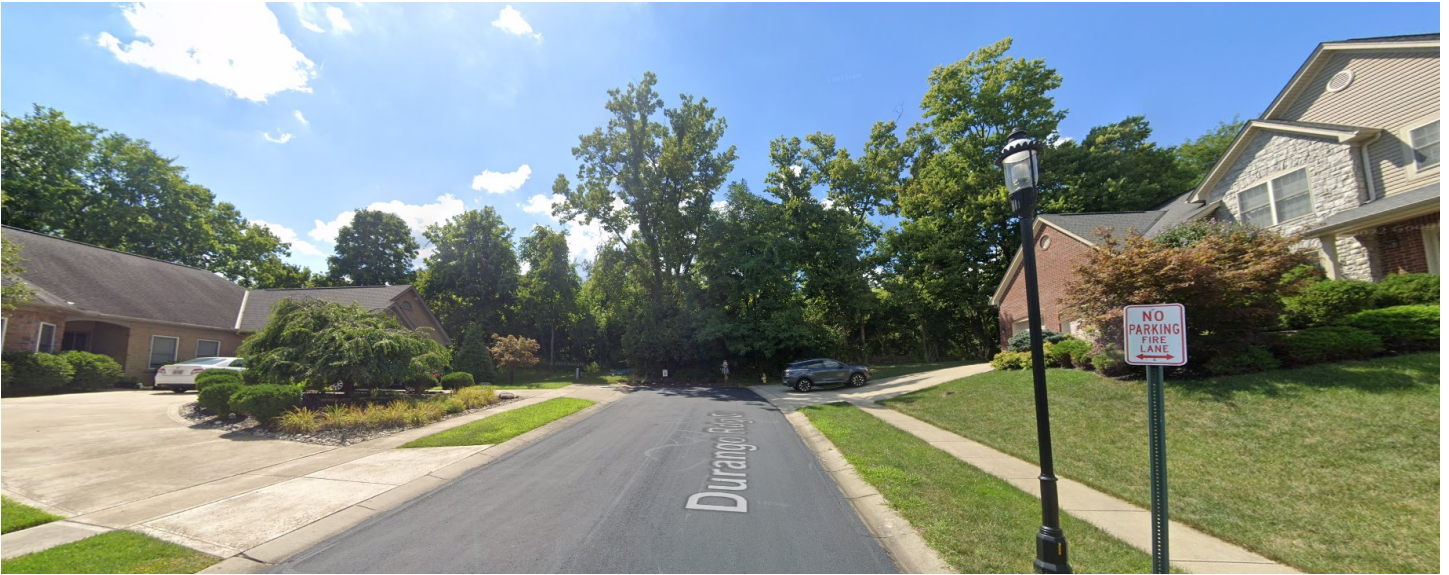
View of site looking west from Durango Ridge stub (google streetview)
